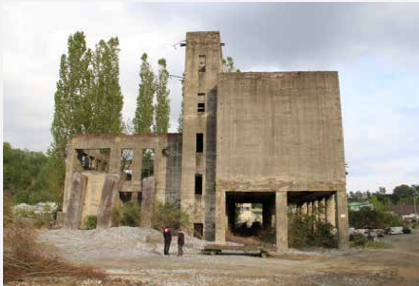
Fig. 3: Gravel crusher in its current condition © Mauthausen Memorial, Photo: Bernhard Mühleder
